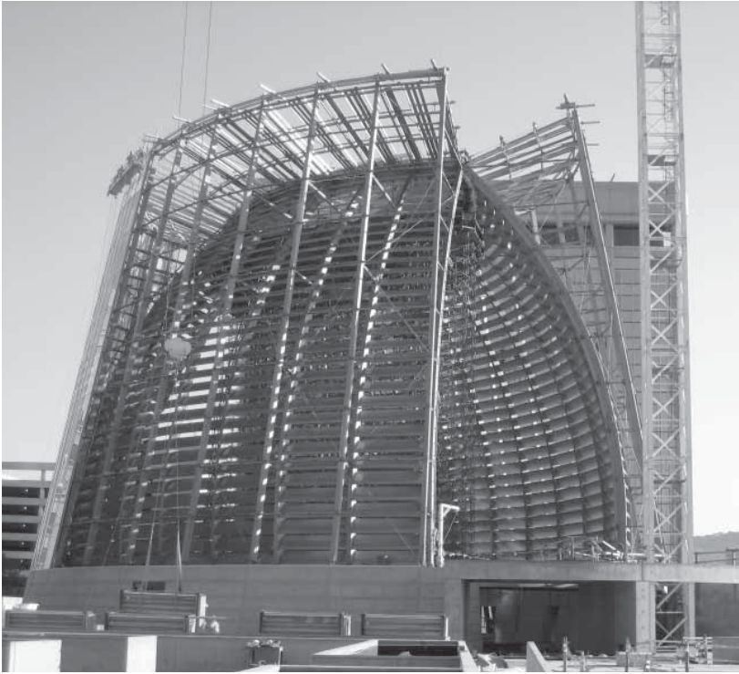
Cathedral of Christ the Light in Oakland, CA is unlike any structure in the world. The inner chords are made with (26) 10 3/4" curved glulam ribs, roughly 100' in length and varying in depth from 30" at the base to 19 1/2" at the top.
