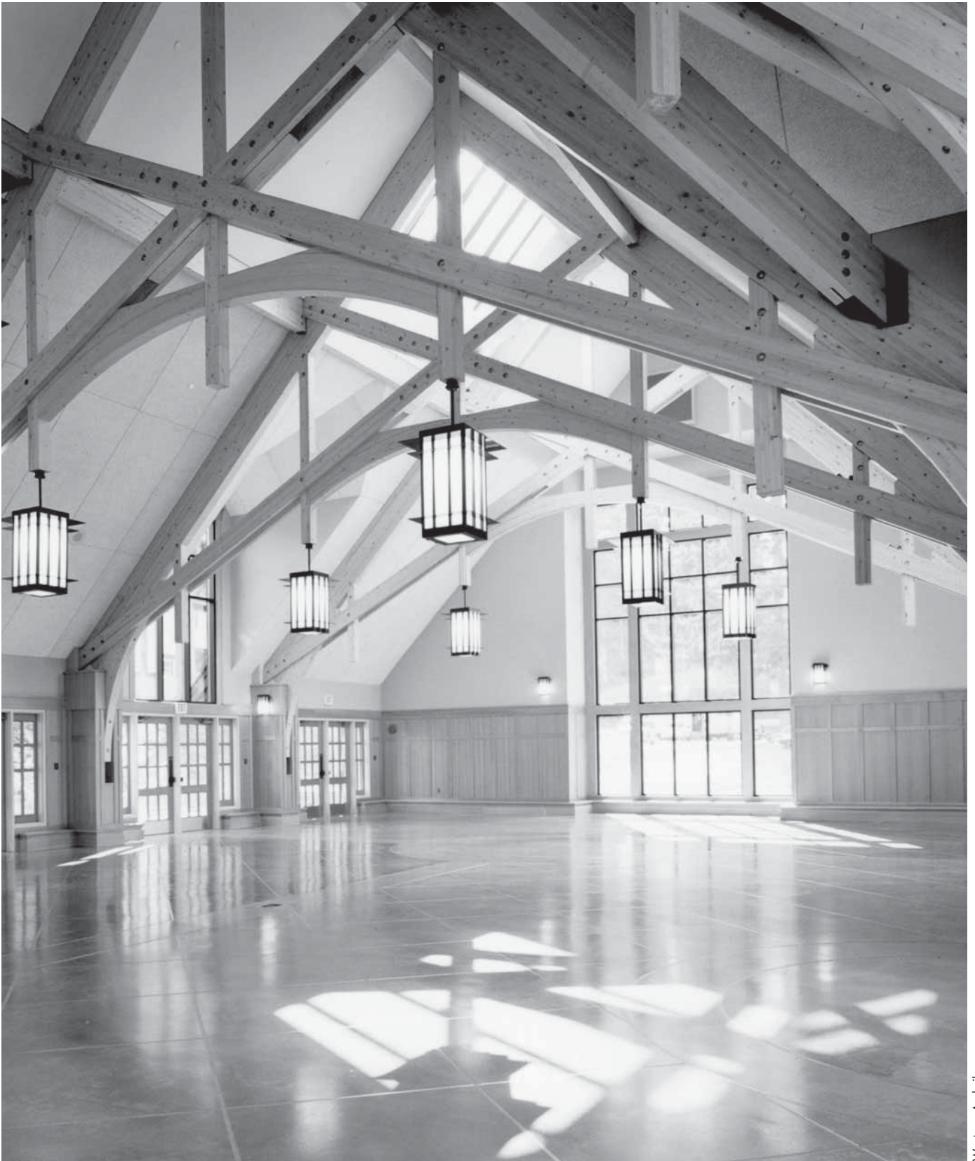
The classic symmetry of these pitched glulam trusses frame the dining hall at Shawinigan Lake’s Marion Hall in British Columbia.
