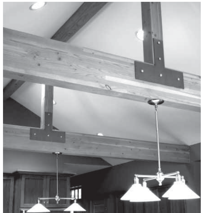
Glulam is available in a range of appearance classifications: framing, framing-L (LVL lams outermost surfaces), industrial, industrial-L (LVL lams outermost surfaces), architectural and premium.
